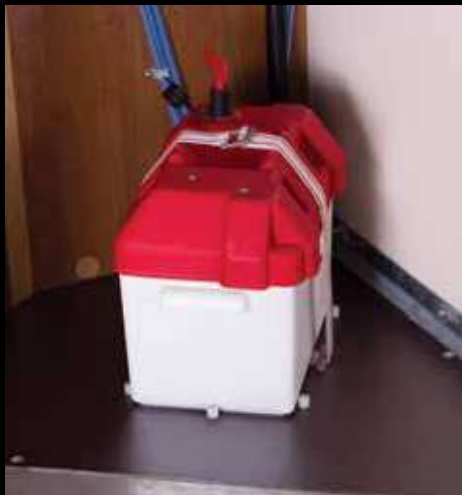
On board 12v electrics
