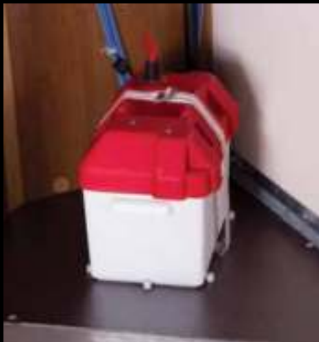
On board 12v electrics
